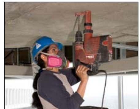
Drilling using a dust cap
