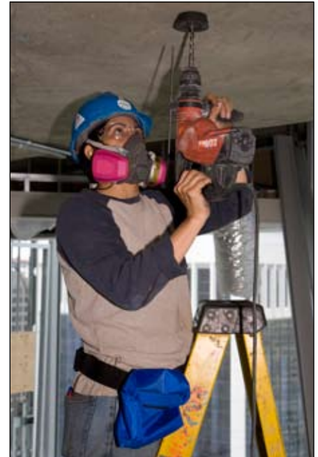
Drilling using a dust cap
